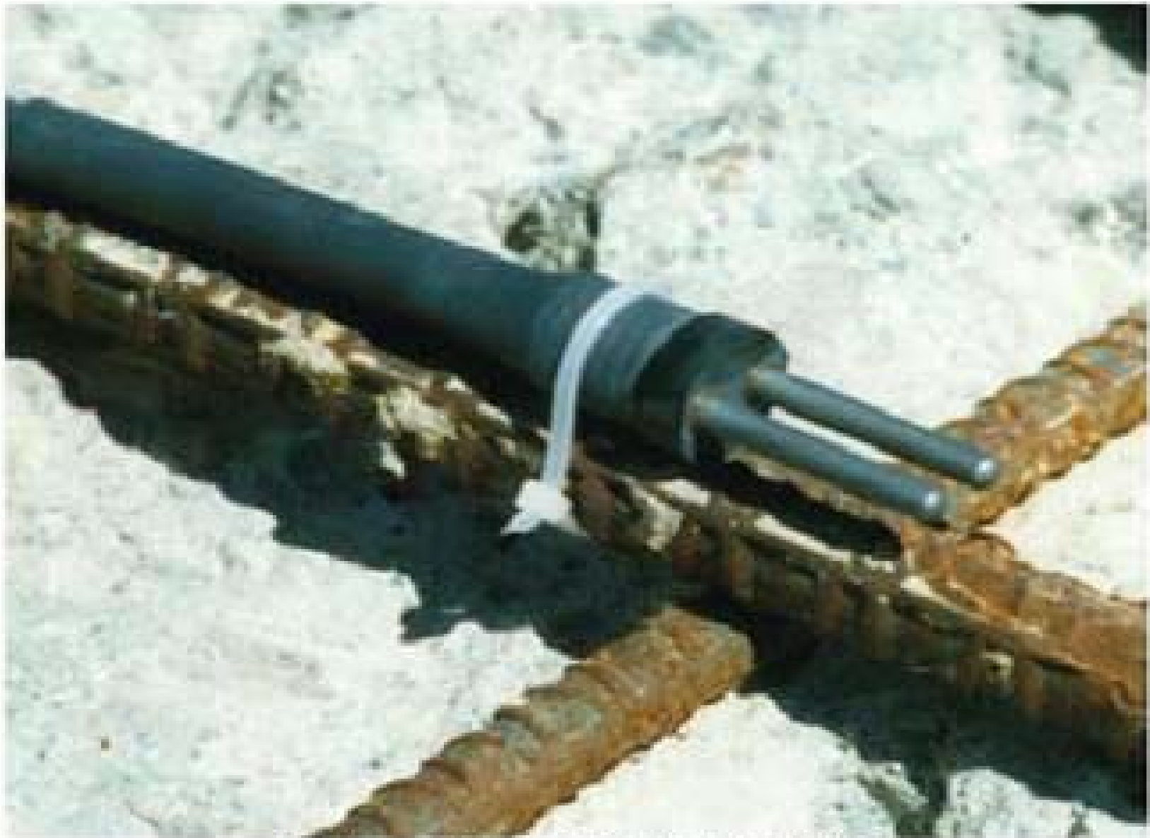
Probe mounted above the rebar Electrode length 1.25" (32 mm)
